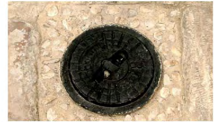
Surface box for a house connection
