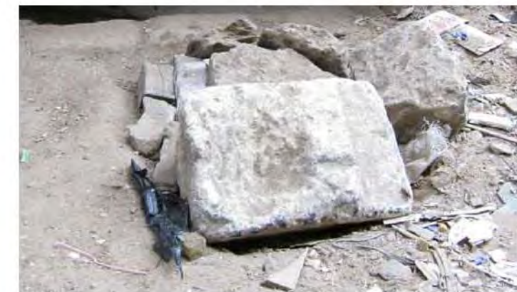
Inspection chamber covered by a stone block
