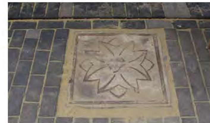
New inspection chamber cover
