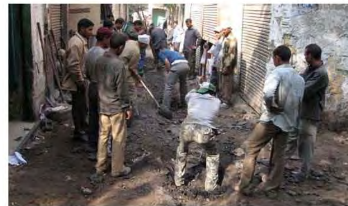
5 Unpaved due to infrastructure improvements
