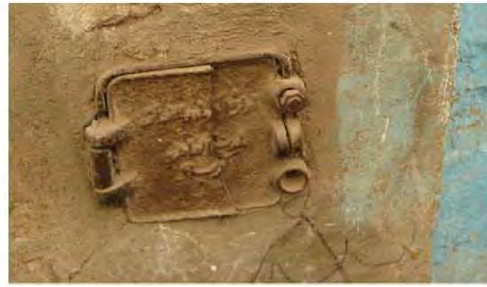
Building connection box with a broken steel cover
