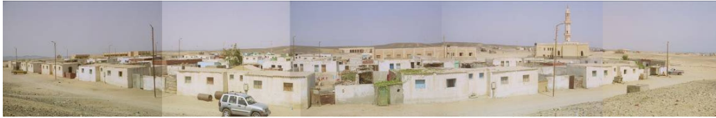
Figure 20 the “Tawteen” houses are made of concrete stones and asbestos ceilings
