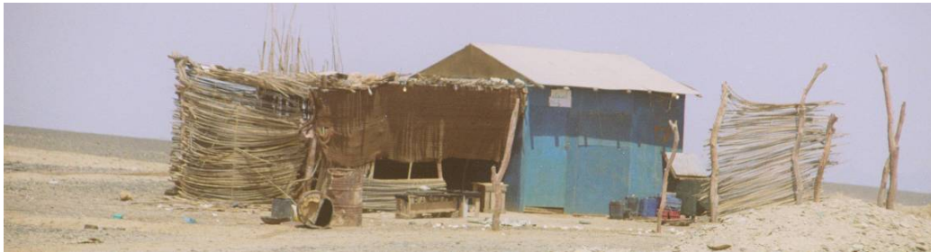
Figure 21 example of the shacks in the village of Hamata, (built by wood, steel and grass-mats)
