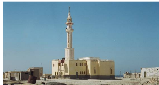
Figure 17 The village main mosque
