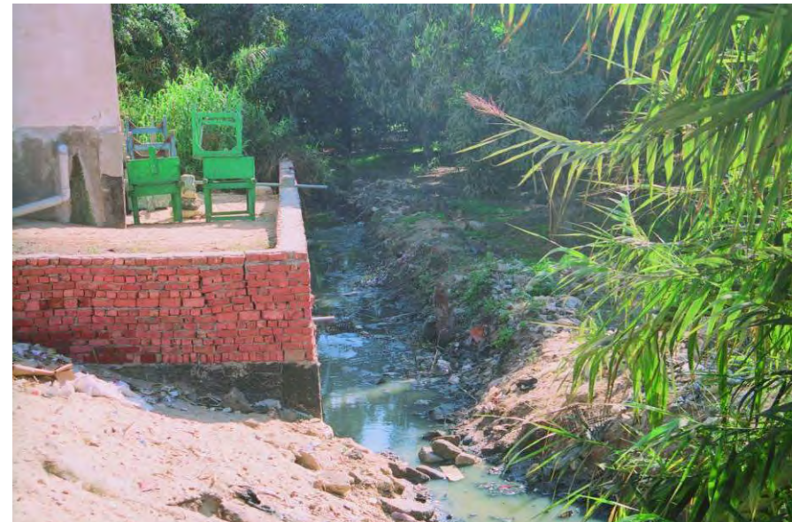
Figure 26 main drainage channel extremely contaminated
