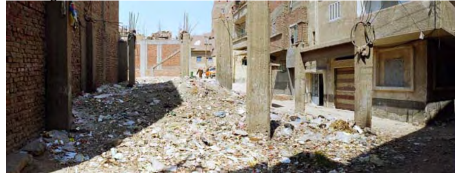
Figure 21 Building without permit
