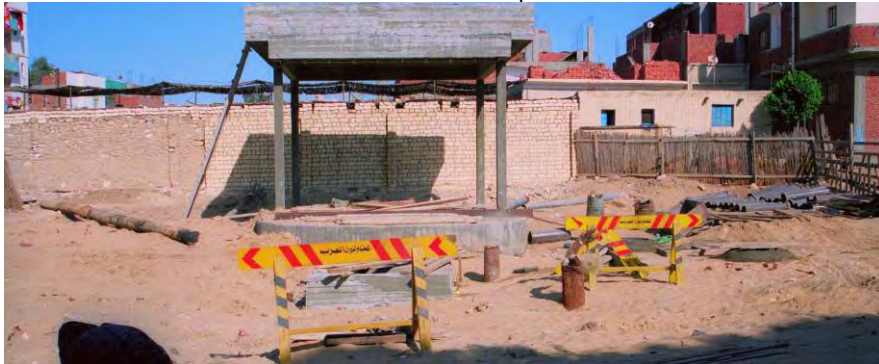
Figure 18 Waste Water Plant is currently being constructed [Jan-06]
