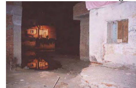
Figure 27 No waste water system
